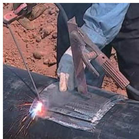
廠外受損管線修復
