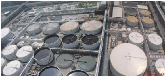
Wastewater Treatment Plant (Before improvement)
