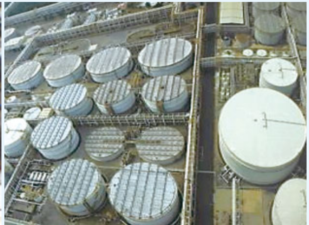
Wastewater Treatment Plant (After improvement)
