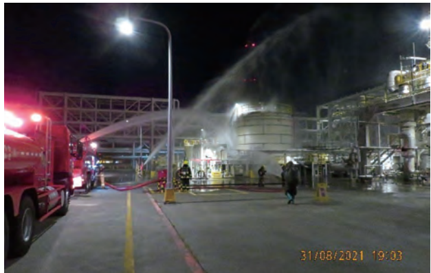
Nighttime toxic chemical leakage response drill
